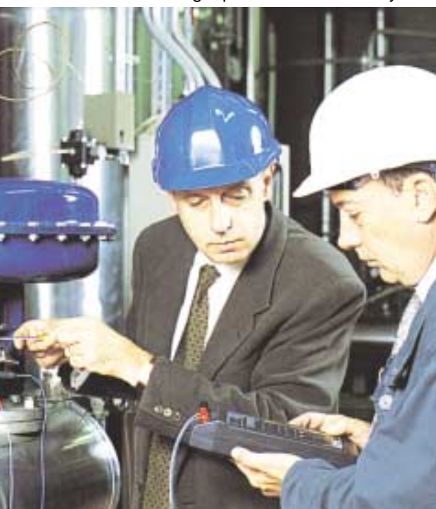
Commissioning a pneumatic controls system
